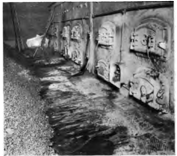
Fig. 5. Safety Tread in Floor of Boiler House.
